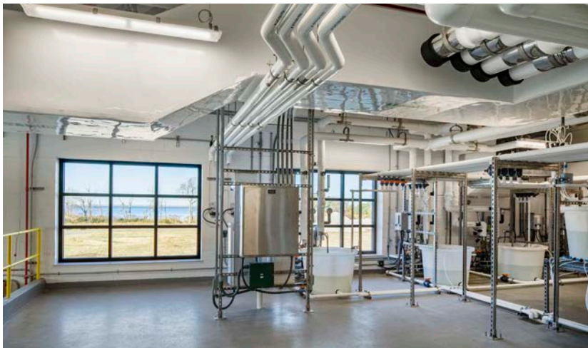
..... Brood Stock Water Controls & Feeding System
