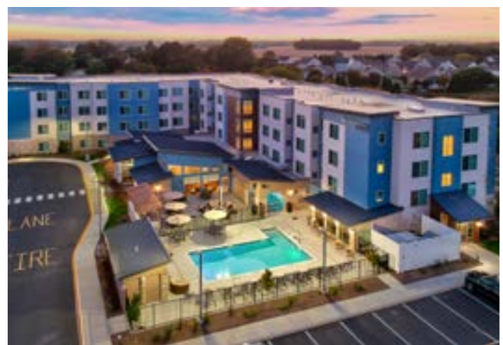
This project was met with tight local height restrictions, paired with ceiling minimums from the brand, and the developer needed a third floor to maximize their investment. The design team worked in tandem with the brand for a six-inch variance per floor to bring the design into local height restrictions.
